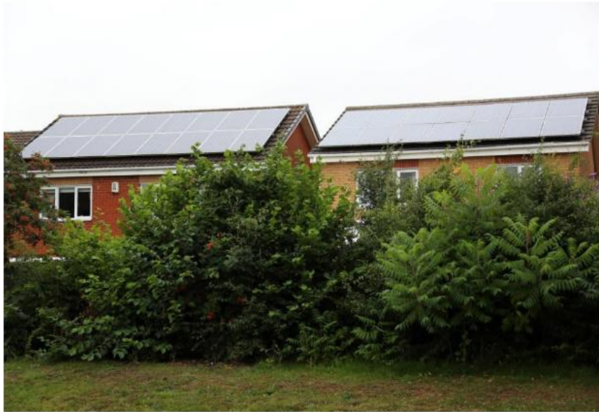
South facing roofs with solar panels
